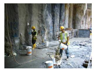
TamPur 100 / Tam Kat 100 is a single-shot hydrophobic polyurethane based on MDI in combination with polyether polyols and an amine based catalyst. The system only reacts when it comes into contact with water, producing a rigid polyurethane foam.
